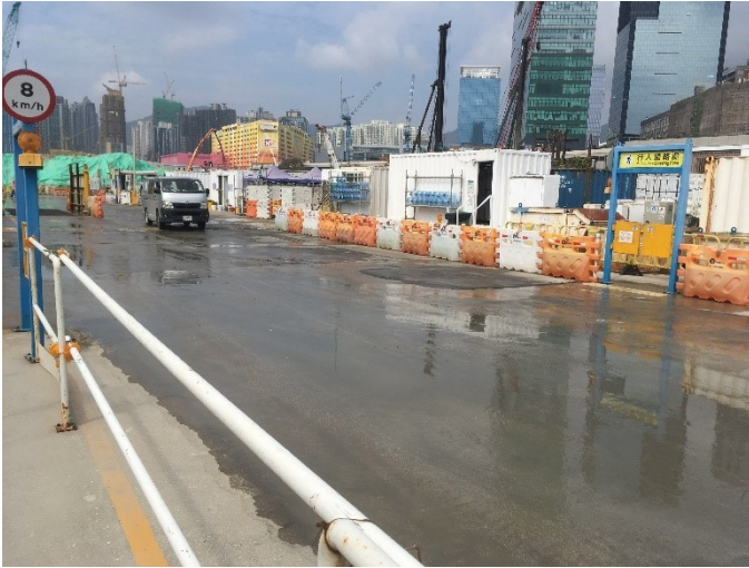
Photo 4 – Watering of main haul road
