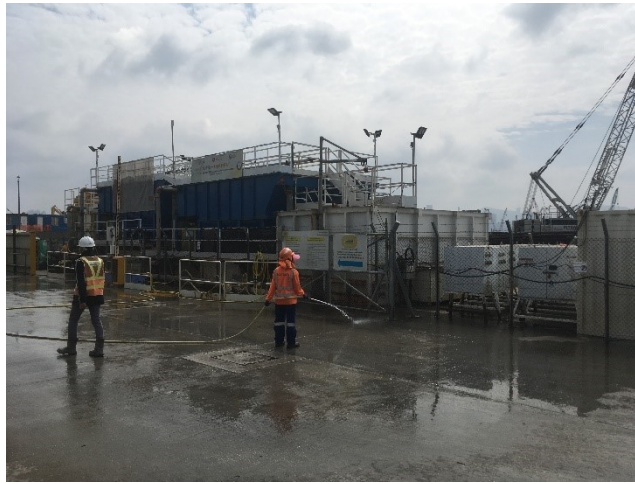
Photo 6 – Watering of main haul road
