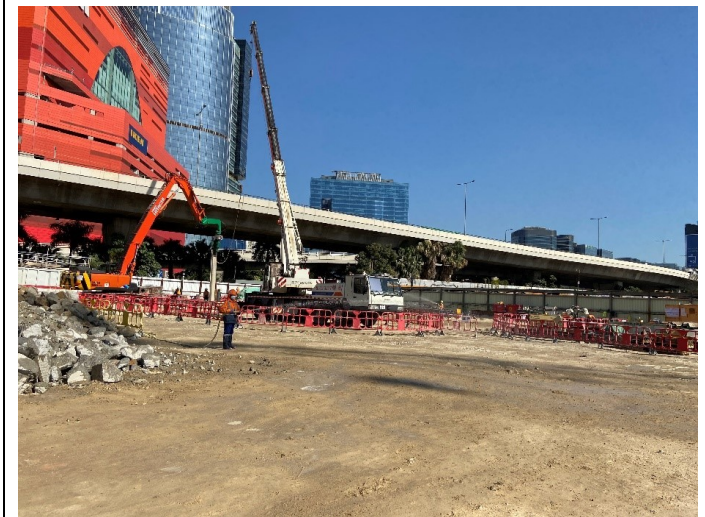
Photo 10 – Watering of unpaved road
