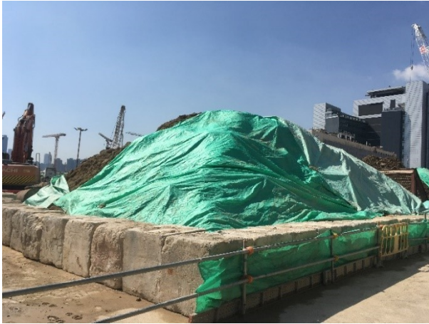
Photo 3 – Tarpaulin covering of open stockpile
