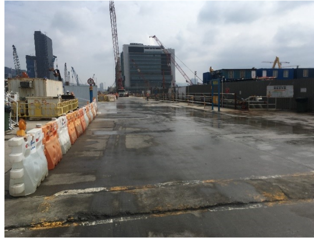
Photo 5 – Watering of main haul road
