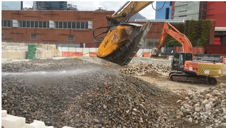
Photo 6 – Water spraying during dusty activities
