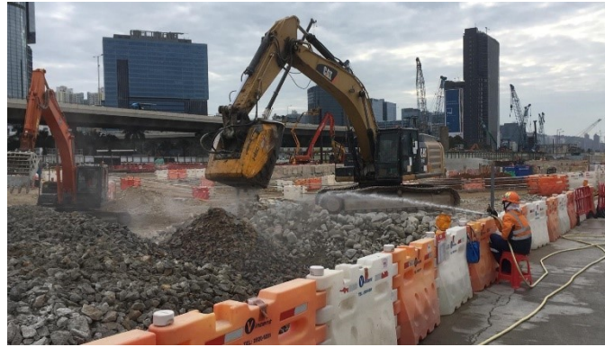
Photo 6 – Water spraying during dusty activities
