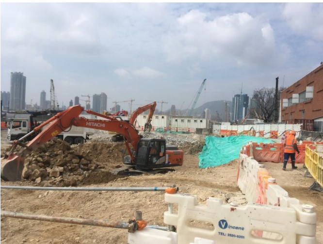
Photo 8 – Tarpaulin covering of open stockpile
