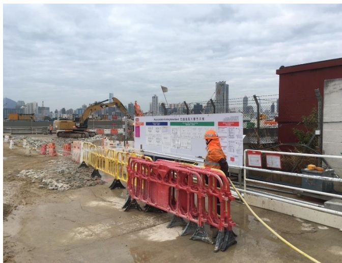
Photo 9 – Watering of unpaved road
