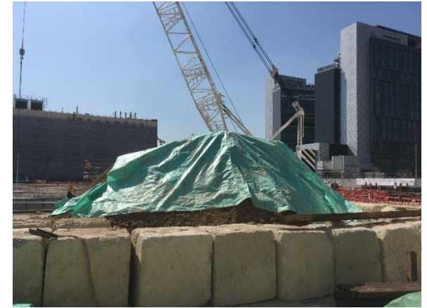
Photo 5 – Tarpaulin covering of open stockpile
