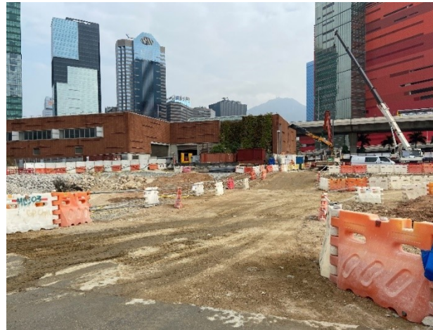
Photo 10 – Watering of unpaved road
