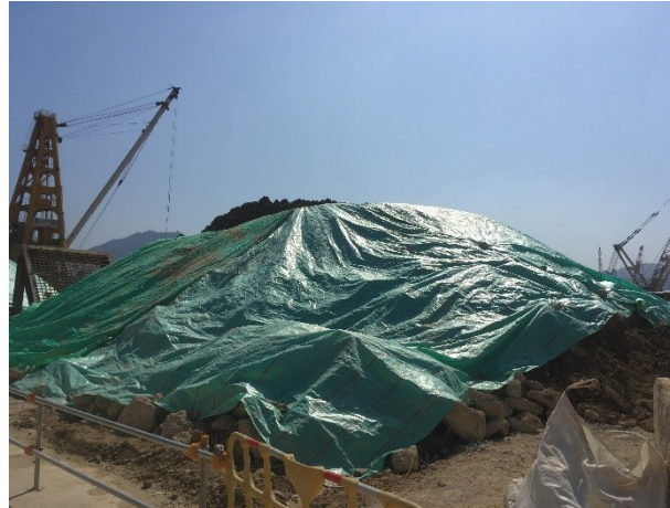
Photo 4 – Tarpaulin covering of open stockpile
