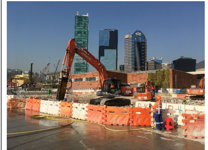
Photo 7 – Water spraying during dusty activities
