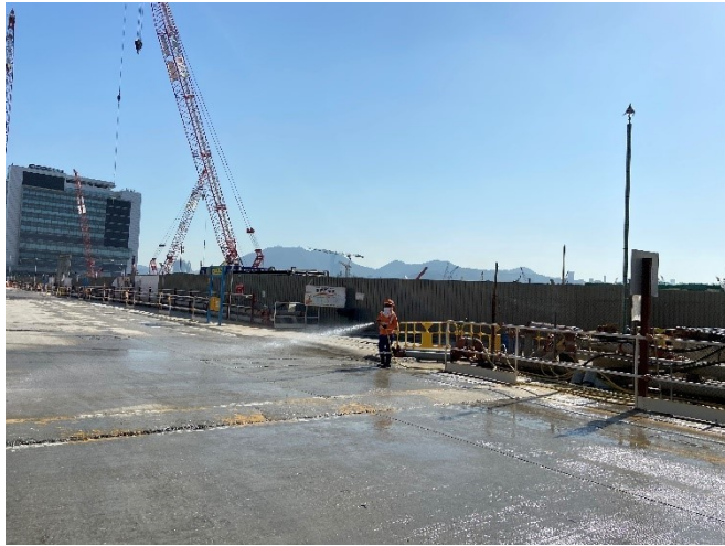
Photo 5 – Watering of main haul road
