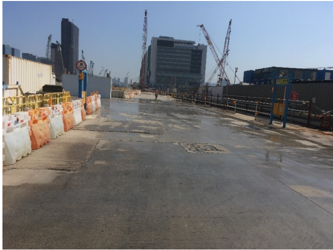
Photo 6 – Watering of main haul road
