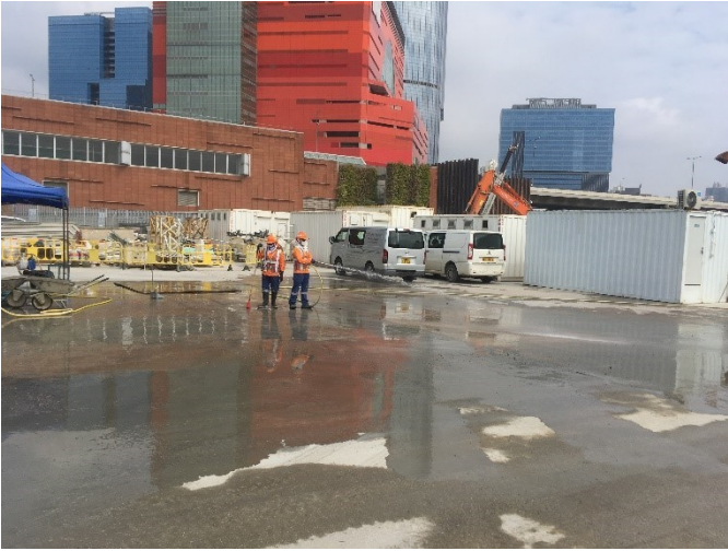
Photo 5 – Watering of main haul road
