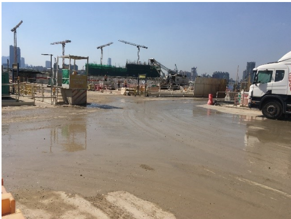
Photo 6 – Watering of main haul road
