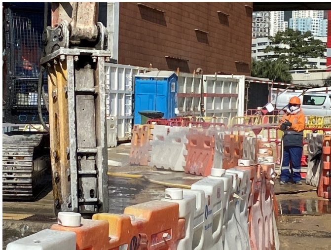
Photo 8 – Water spraying during dusty activities
