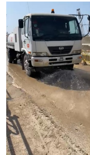
Photo 8 – Watering of main haul road
