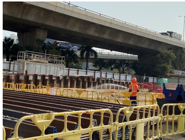
Photo 9 – Watering of unpaved road
