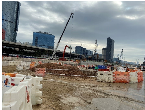
Photo 7 – Watering of unpaved road
