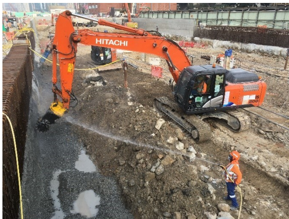
Photo 9 – Water spraying during dusty activities
