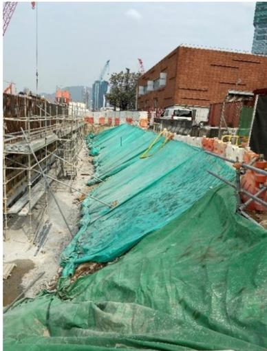
Photo 8 – Unpaved area was covered by impervious sheets
