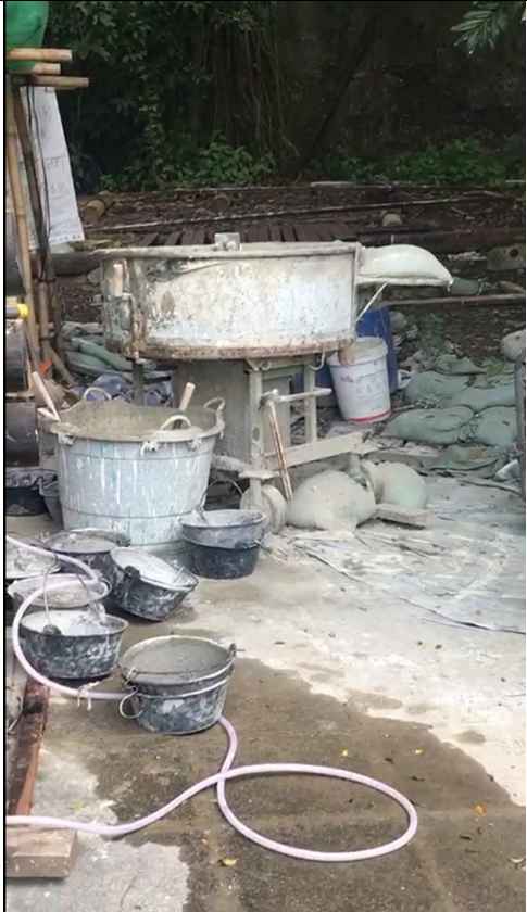
Video Screenshot 1 - Cement mixing carried out by the worker of Temple renovation work
