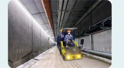
space underneath the tunnel carriageway as a service gallery to house the E&M facilities, drainage and fire services for the tunnel. This enables tunnel operators to carry out inspection and maintenance works at any time without affecting the tunnel traffic. Electric vehicles are provided ins the service gallery to facilitate inspection and maintenance works by tunnel operators and allows firefighters to quickly reach the fire location.
